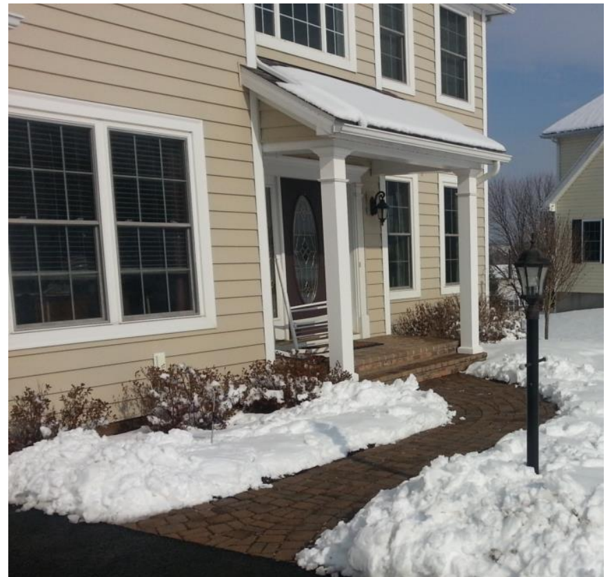
Residential Microgrid Test Site, Lewisburg, PA USA
